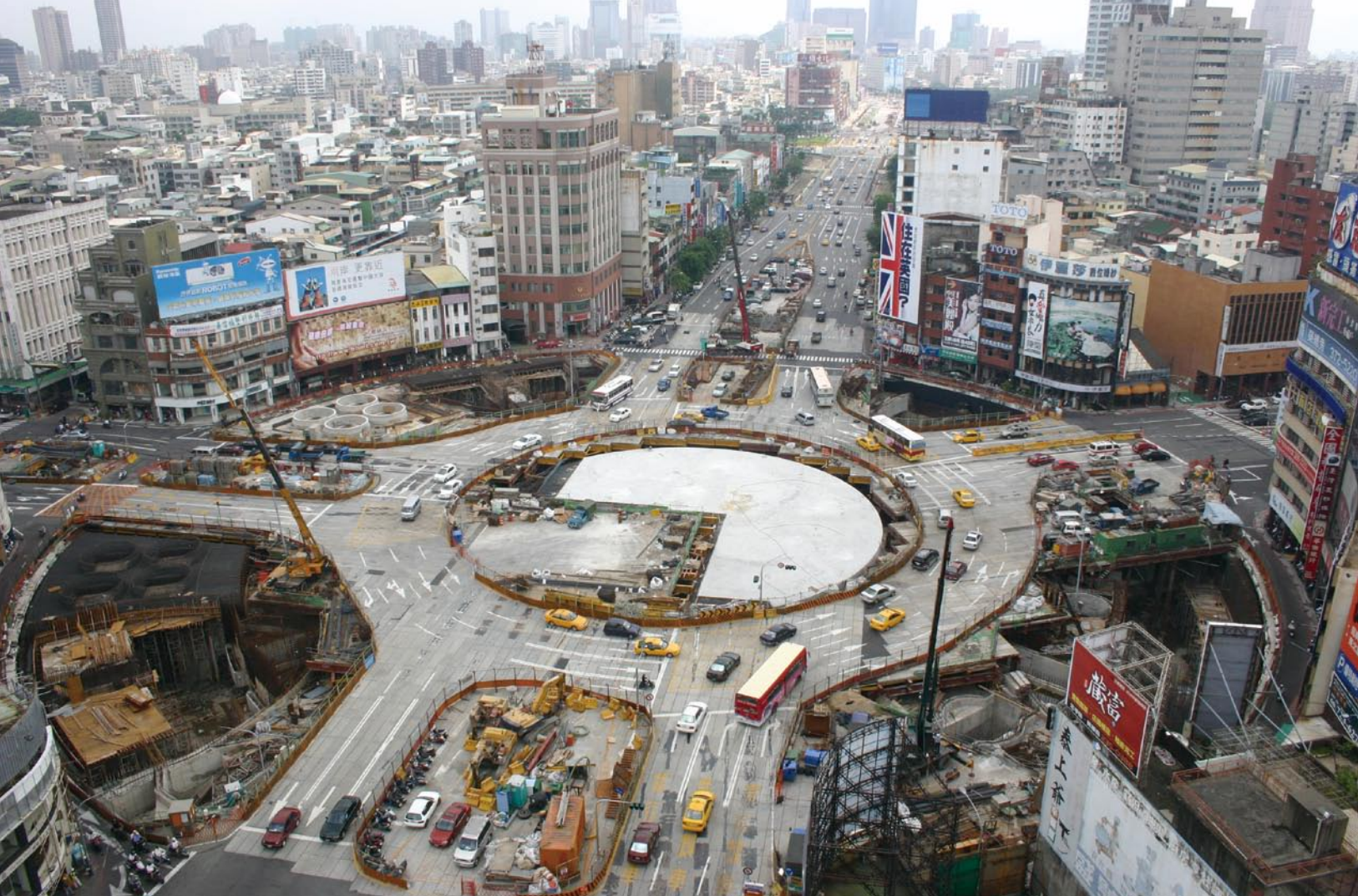
Construction on the intersection is proceeding on schedule.
