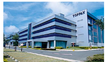
The newly built Toppan CFI (Taiwan) factory
