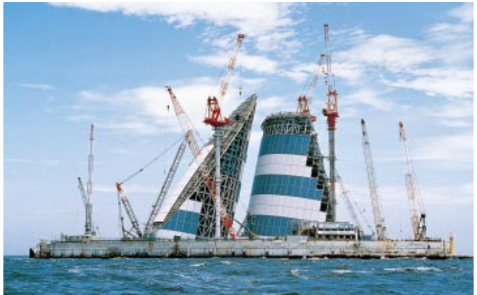
Photos supplied by TRANS-TOKYO BAY HIGHWAY CORPORATION
