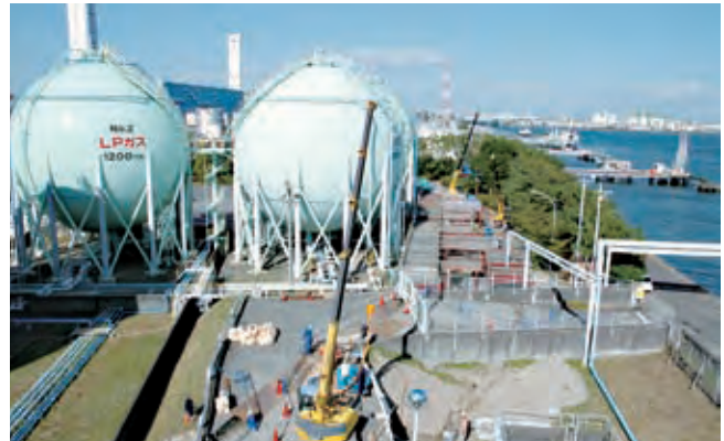
Construction work to prevent coastal erosion at the LNG Terminal (Constructed by Chemical Grouting Co., Ltd.)
