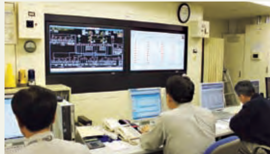
Building management work
