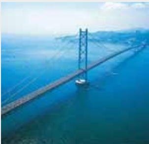
Akashi Kaikyo Bridge
