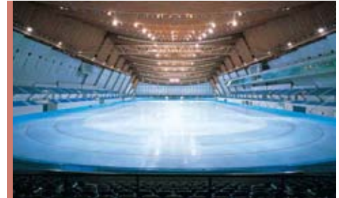
Nagano Olympic Memorial Arena
