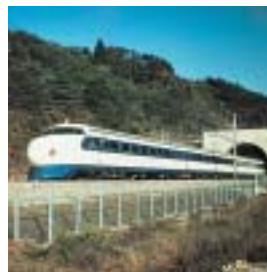
1963 New Tanna Tunnel
