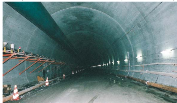
Progress is being made in the underground tunnel construction work.
