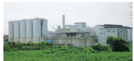
View of the METAKLES facility
