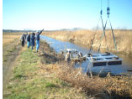
Installation of rafts using a crane
