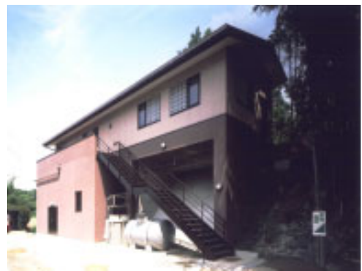
Protective structure for the Kitora tumulus
